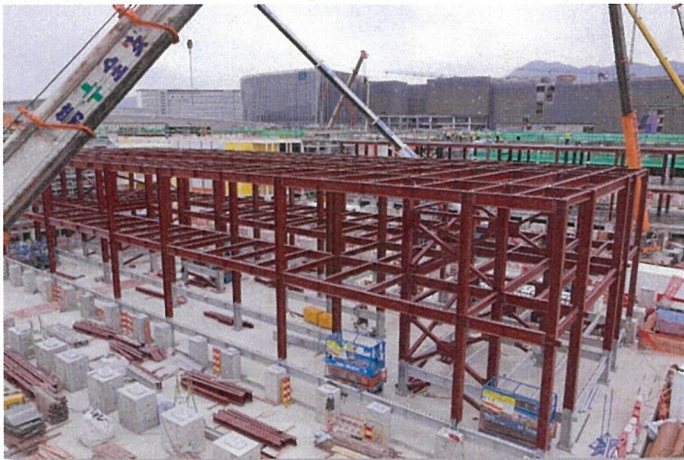
Medical Block & Ward Block Common Area Pre-fab Steel work
