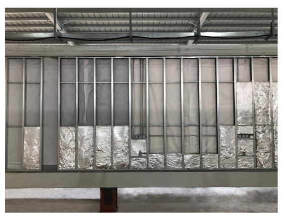
轻钢龙骨复合墙体地面预拼,整体安装 Light steel keel composite wall and ground pre-assembled, overall installation
