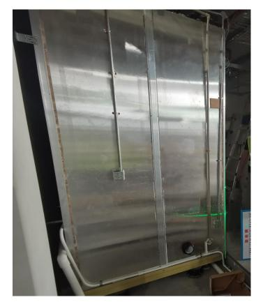
整体卫浴金属一体板 Whole bathroom metal integrated panel
