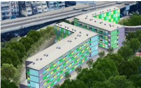
Transitional Homes at Yen Chow Street in Sham Shui Po (4 Storeys)
