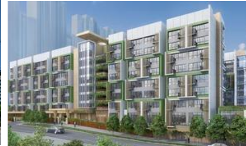
Residential Care Homes for the Elderly ("RCHE") in Kwun Tung North (8 Storeys)
