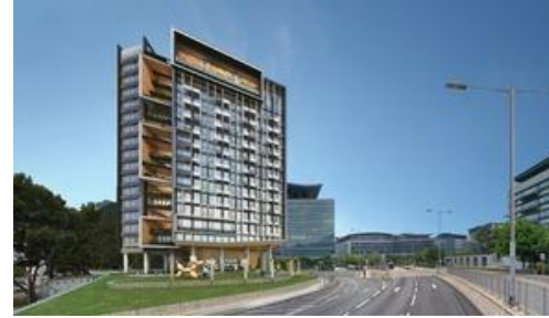
InnoCell at Hong Kong Science Park (15 Storeys, 59.2m(H))
