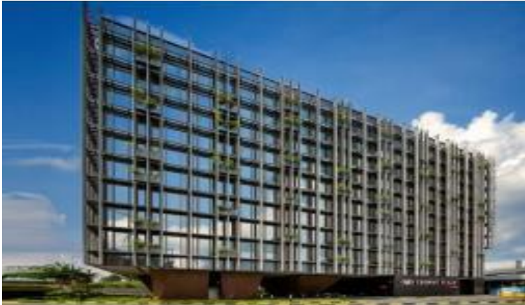
Crowne Plaza Hotel Extension (10 Storeys)
