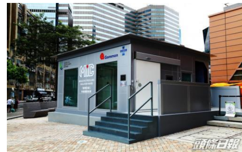
MiC Negative Pressure Isolation Ward (Prototype) at Zero Carbon Park, Kowloon Bay
