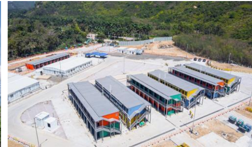
Temporary Quarantine Facilities at Penny's Bay
