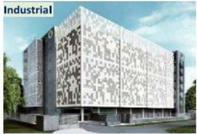
Global Switch Data Centre (5 Data Floors)
